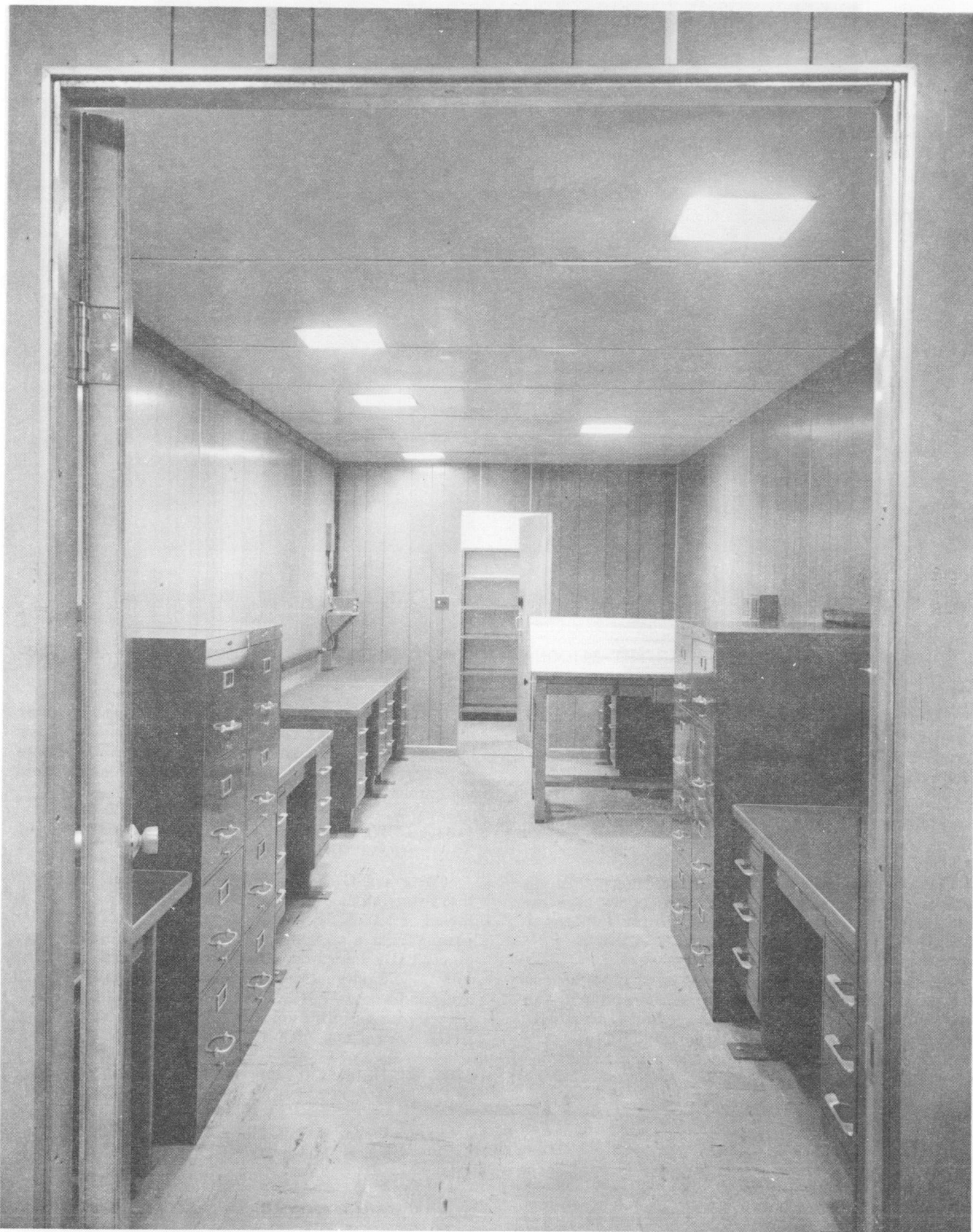
Figure 1-31. Receiving Central Group OA-4966/TSR-1 (RG1, Equipment Installation)
