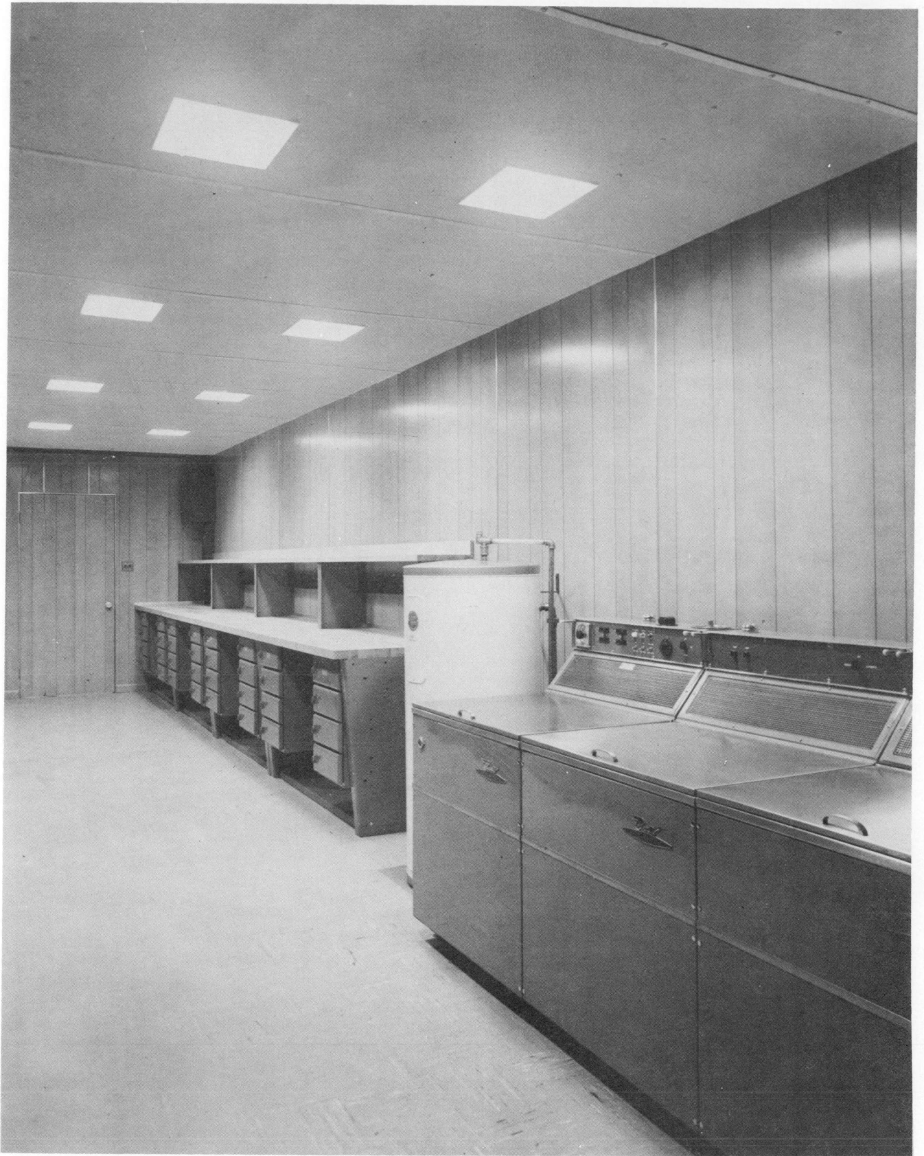
Figure 1-33. Maintenance Equipment Group OA-4967/TSR-1 (RH1, Left Side Equipment)
