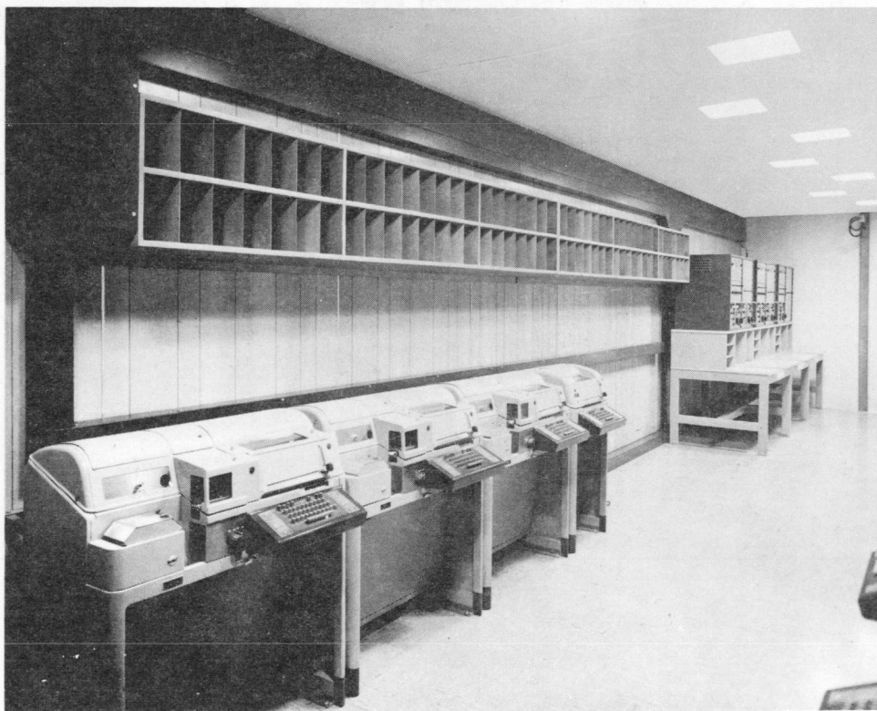
Figure 1-28. Control Monitor Group OA-4950/TSR-1 (RF2, Left Side Equipment)
