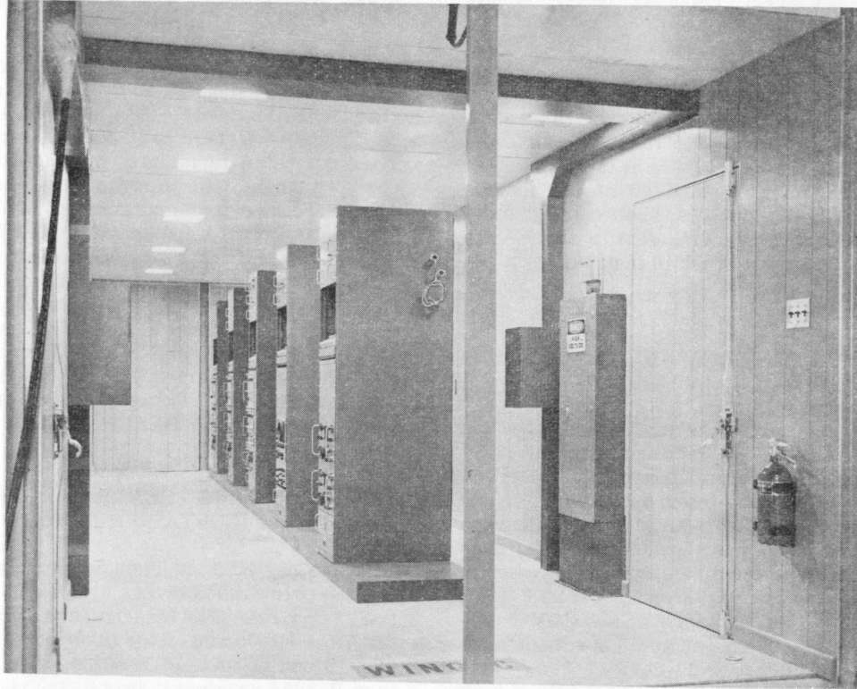
Figure 1-16. Receiving Central Group OA-4939/TSR-1 (RC1, Equipment Installation)
