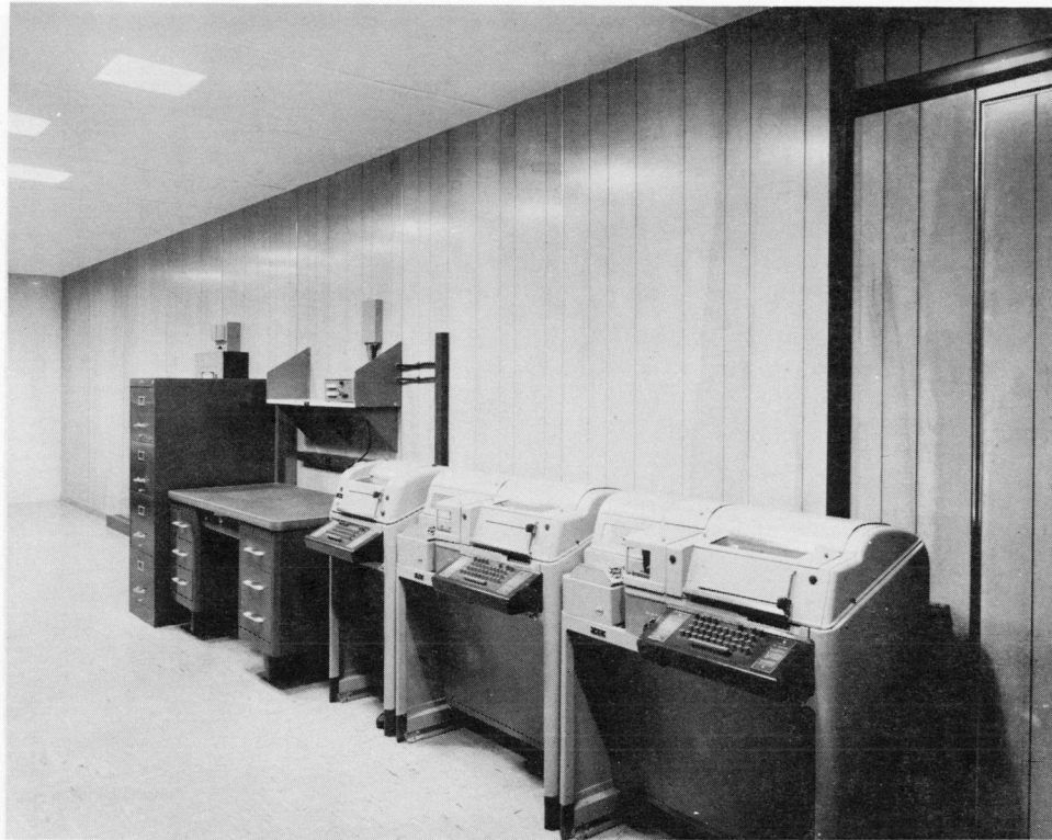
Figure 1-29. Control Monitor Group OA-4950/TSR-1 (RF2, Right Side Equipment)
